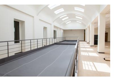
Horizontal firecurtain is ideal for the fire compartment of large openings up to  $12 \times 3$  m (max  $36 \text{ m}^2$ ). It can be installed on the ceiling and closes automatically in case of fire.
